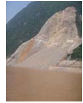
Landslide in reservoir
