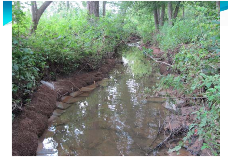
Stream bank stabilized with protected toe
